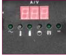
System status and error indicator lights.
